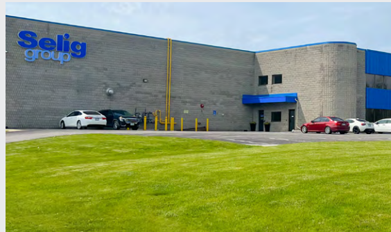
BRADFORD, CANADA: Opened in 2022, Bradford is Selig's Lift'n'Peel Center of Excellence.
