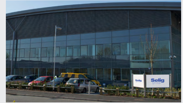
SLOUGH, U.K.: Opened in 2012, Slough is our international headquarters, producing a wide range of sealing solutions.
